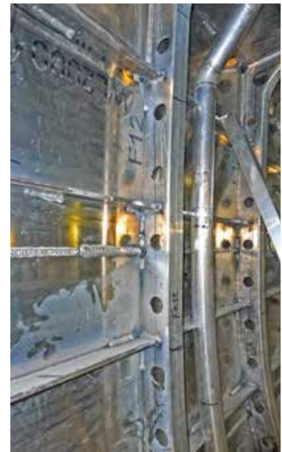
Right: The strong frames with strapping and relief holes.
