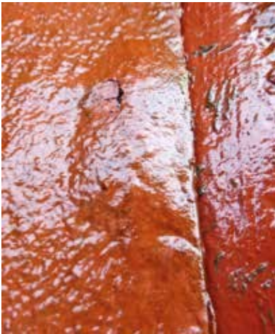
This bubble is evidence of coating detachment. The cause must be checked.
