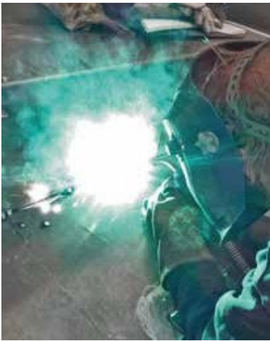
The welding takes place in "pilger" steps to keep the delay within limits.
