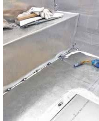
The re-sanded seam is prepared to weld the next step.
