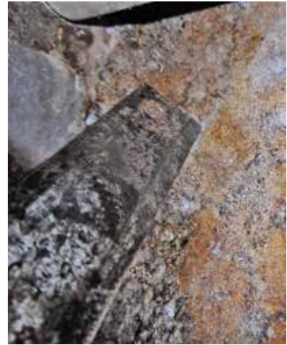
This coating in the water tank must be removed so that any corrosion that may be present underneath it can be detected.
