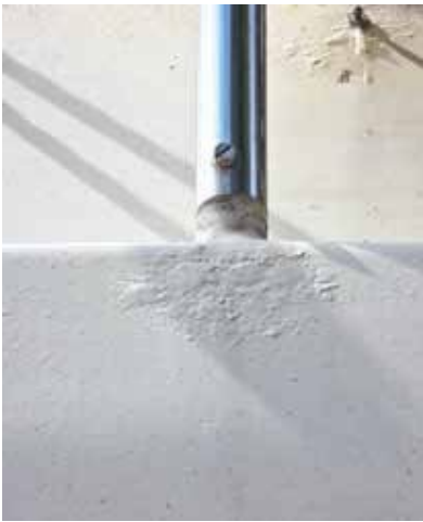
Here, the paint blooms under a railing support made of stainless steel; slight corrosion under the paint would be possible here.
