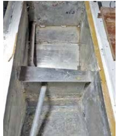
Lead bars were stored in this ballast room. After leakage, considerable pitting corrosion occurred.
