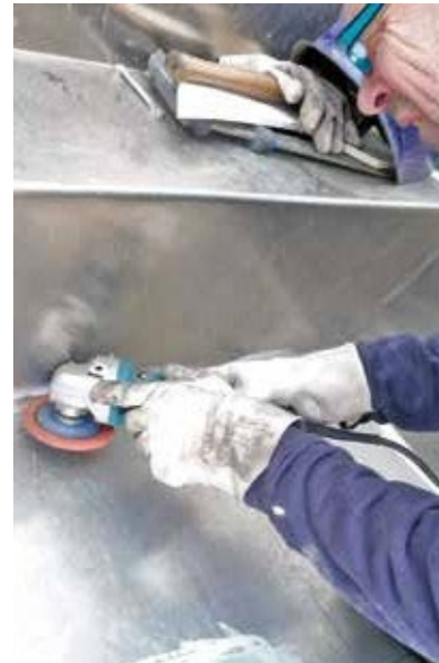
All seams are sanded in between before welding continues in "pilger" steps.
