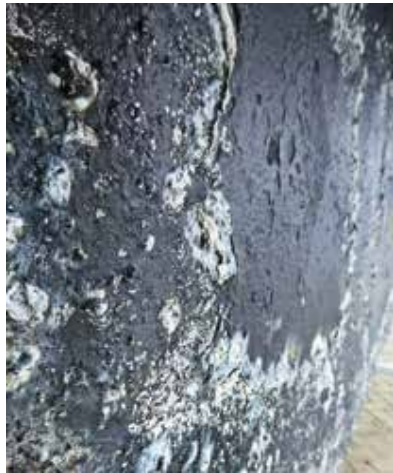
Aluminium oxide blooms beneath the paint, a sign of more serious corrosion damage.
