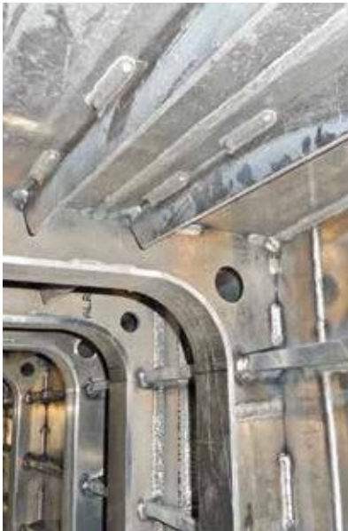
The deck knee with its relief hole is integrated into the bulkhead frame.
