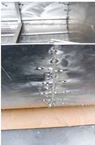
At the stapling points it can be seen where the studs were fastened to align the plates and keep them straight.
