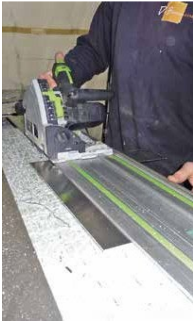
Aluminium cutting of flat material is done with a circular saw.
