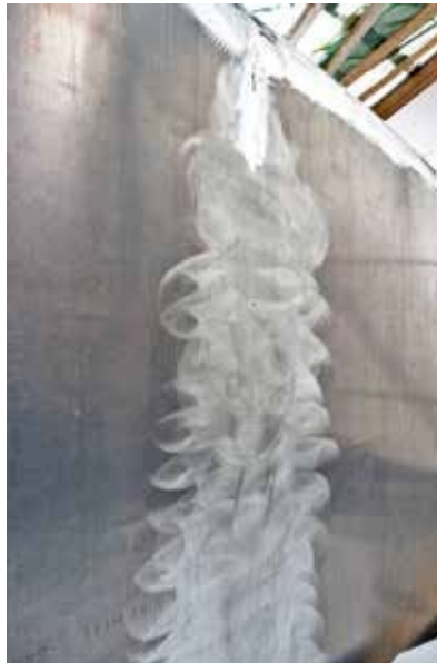
After sanded, the weld seam and the stapling points are no longer visible.
